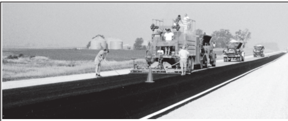
Slurry / Micro Surfacing
